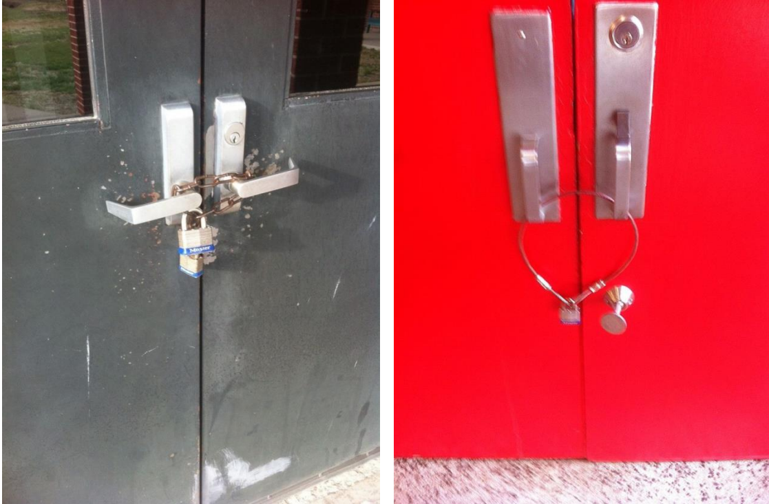
Figure 16: Doors locked in various manners.
