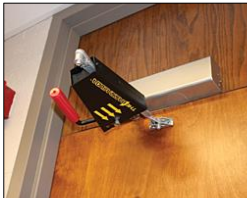
Figure 12: Crank-type Door Closer Restrictor by Bilco Corporation in installed position.
